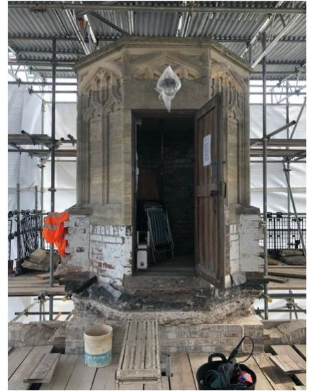
could be felt in the roof. Additionally, the ends of the steel beams were revealed to be corroded right through. The structural engineers took rapid action to install a crash floor beneath the roof and brace the tower with a scaffolding cage. This was dangerous work and the professional advice was that the roof and part of the top of the tower was ready to collapse. Such a catastrophe would have brought down more than 50 tonnes of rubble and steel into the sanctuary and through the roof.
