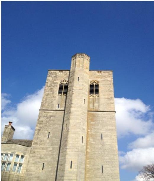
Back in 2015 it was discovered that the stonework at the top of the tower was distorted and an estimate that the cost of repair might be £60,000 was provided. [Historic England](#) underlined the critical situation by placing the Church on the 'Heritage at Risk' register.
