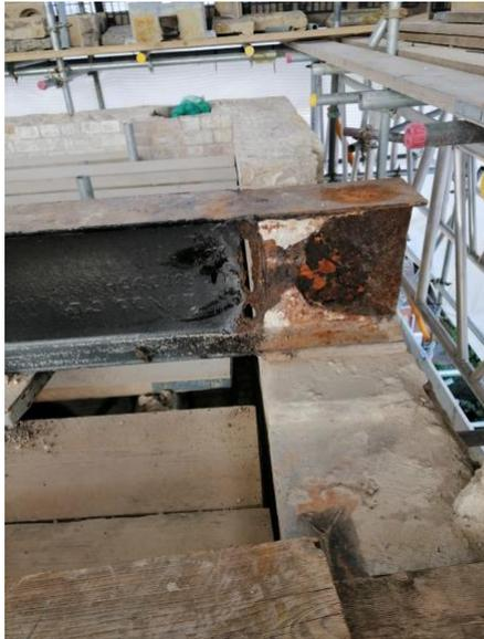
Work to reveal the extent of the damage to the tower roof began in July 2019. As more of the roof was revealed the extent of the problems increased. The concrete roof slab was cracked through in several places and the reinforcing mesh had clearly broken down to the extent that when the asphalt was removed movement
